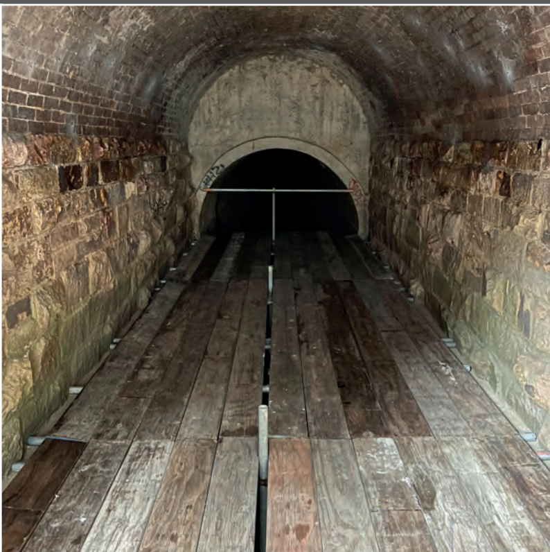
Heritage Culvert, Wooloowin
